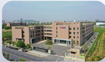
R&D Center 4 professional lab and production area: 70,000 m 2
