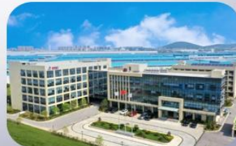
Management & Sales & HR & office building
